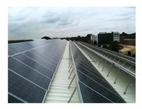
Sunlink Energy Adjustable Tilt Solar Racking System is applicable to install the usual framed module to tilt a certain angle with the roof. The solar system can be a fixed angle or adjustable such as 10~15 deg, 15~30 deg
