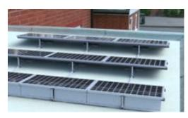
engineered solution that secures the array without damaging the flat roof. It is compatible with the usual framed photovoltaic modules and typically does not require roof penetrations. Made from lightweight and strong
